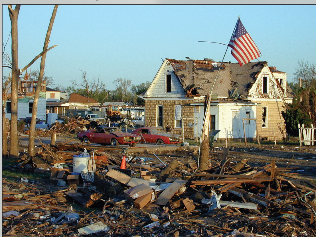
An American flag flies over the debris left in the wake of a tornado which struck Hoisington, Kansas. More than 400 homes were damaged or destroyed. (photo by Dave Saville/FEMA News)
