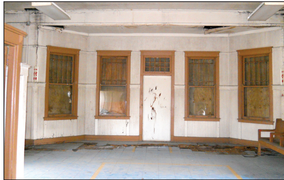
A bay window section of the Durant ICRR Depot waiting room fronts on Highway 12, which is Mulberry Street, in the heart of the Durant commercial district. Renovation plans detail a restoration of the original woodwork and plastered walls in this main compartment of the North Building. The original ticket windows will be retained as partitions between refurbished office spaces and a mini-kitchen will be built next to the central meeting room.
