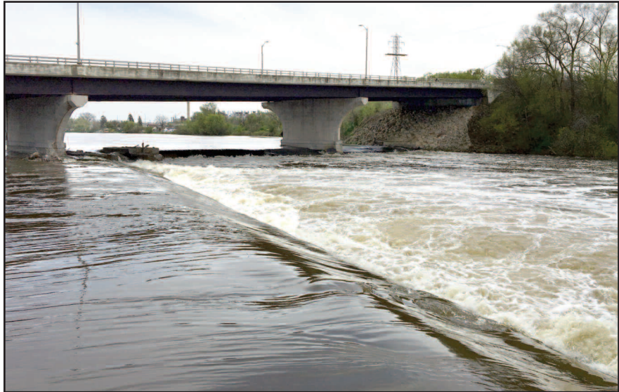
Janesville's Monterey Dam is scheduled for removal in early 2018. (Photo by Jason Francis)
