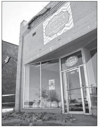
The former home of Tiara's & Tadpoles is having issues with its crown. Caution tape was placed in front of 224 E. Main Street to protect pedestrians from falling bricks which came loose from the top of the building.
