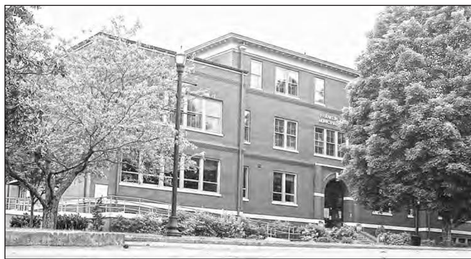
The Blue Building has been vacant since November 2009. Efforts to find a tenant or buyer for the property have failed thus far.
