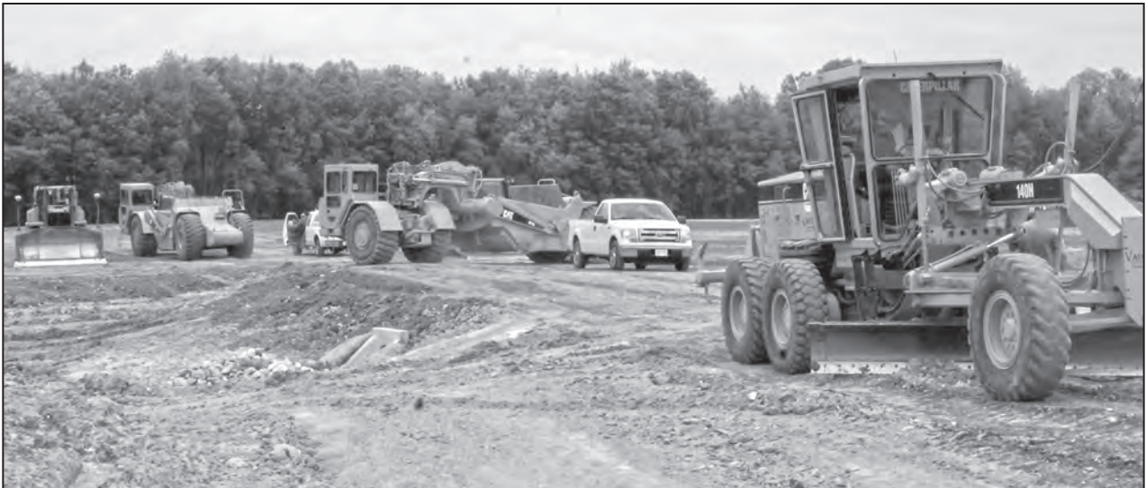
Heavy equipment operators are working to get 700,000 square feet pad ready at Mt. View Industrial Park in Morrison. The work will allow an industry to start construction immediately if this site is selected for development.
