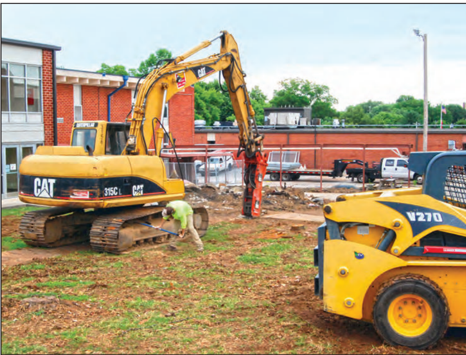
Construction is under way at Bobby Ray Memorial Elementary.
