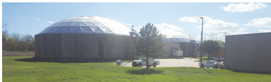
Del City is undergoing a $21 million overhaul of its wastewater plant. The project will bring the facility into compliance with Oklahoma DEQ standards -Provided Photo
