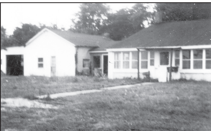
Jenk's Pizza location before remodeling began.
