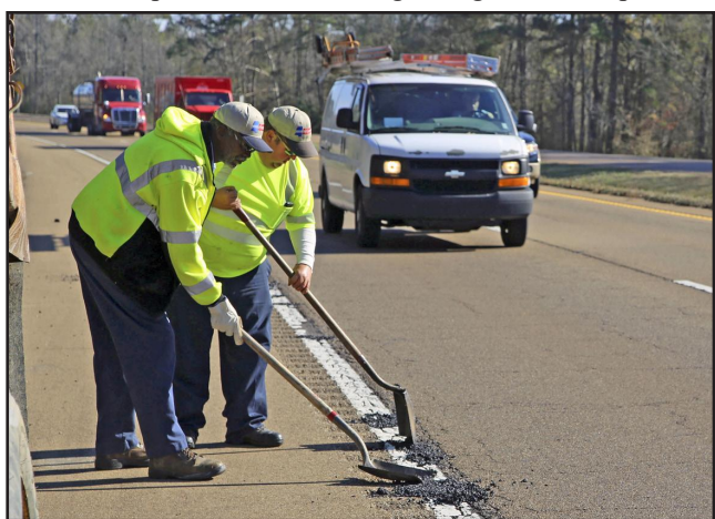
Simpson County maintenance crews patch pot holes as traffic flows by. (Photo by MDOT)
