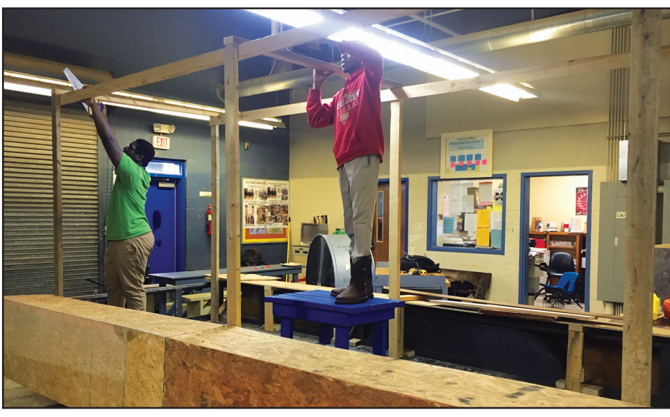
Holmes County Career and Technical students Lathell Bankhead (at left) and Jarvis Mitchell make progress on the framework of the school's float to be presented at the Lexington Christmas parade set for Thursday, November 29. Deadline for parade entrants is Monday, November 26. (Photo submitted)
