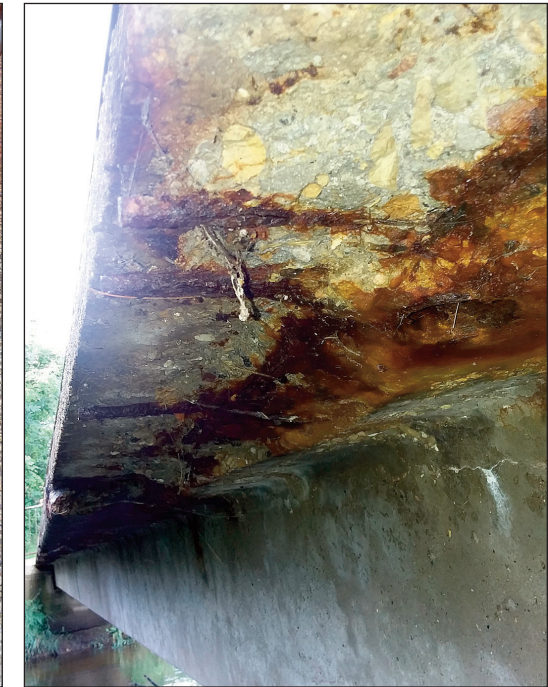
Safety concerns about the Saunders Creek footbridge noted by Edgerton Police Chief Tom Klubertanz included rusting to support railings (left) and damage to concrete on the structure's underside (right), in addition to other issues.
