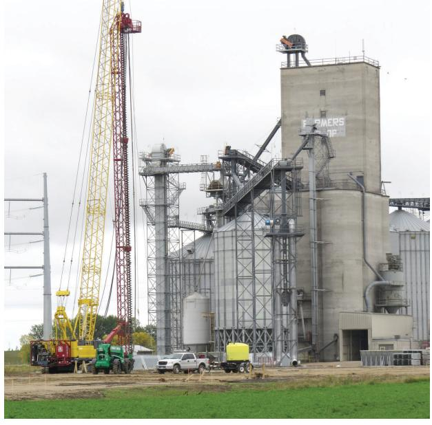
At times the construction of the new bunker was a down and dirty fight with Mother Nature. Heavy trucks slopped their way through mud, slowing progress on the bin site while the calendar kept moving closer and closer to harvest. By September the bunker site was a beehive of activity as foundations were poured and steel erected for the transfer equipment that would move grain from the dump site into the
