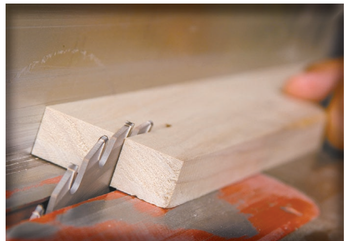
Cutting renovation materials outdoors can minimize dust generated in work areas.
