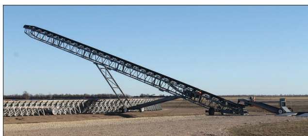
The new MKC grain bunker includes a large motorized grain conveyer belt. The conveyer belt can be moved as needed.
