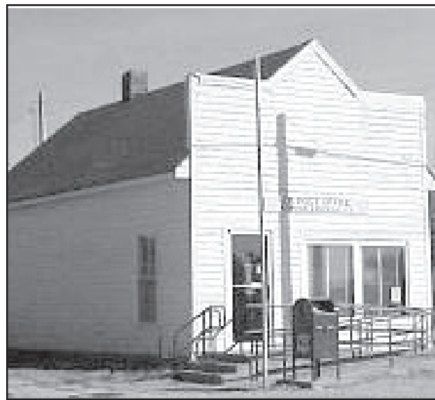
The Raymond post office exterior has not changed much over the years
