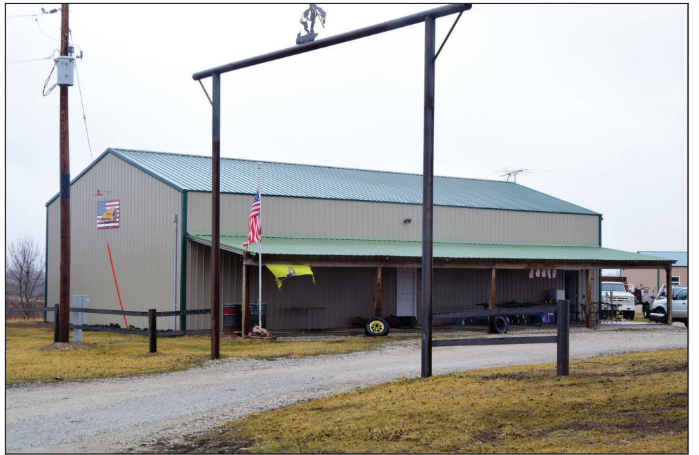
Michael Higday built a machine shed in Athens Township.
