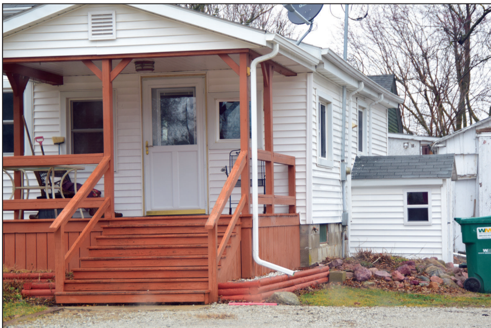
Ervin and Debora Trullinger built an addition to their house and a shed at their property in Tingley.
