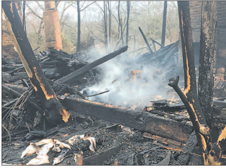
ASHES – Embers still smoldered Monday following a fire that destroyed an unoccupied house on Garlington Street Sunday. Three teens were arrested and charged with arson.
