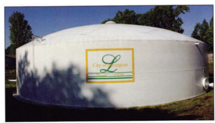
200,000 Gallon Ground Tank
