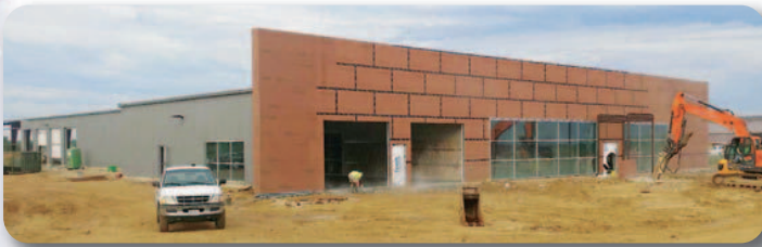
New building now in progress.
