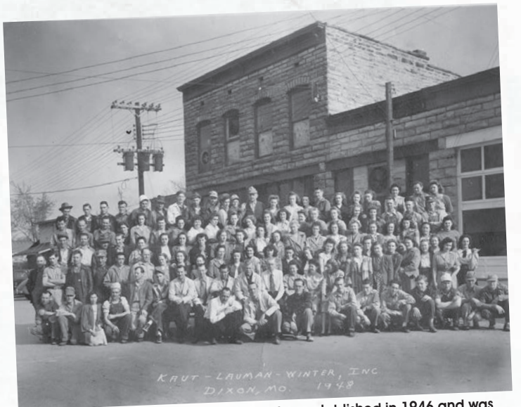
Kaut - Lauman - Winter, Inc shoe factory established in 1946 and was housed in the former American Legion and adjoining buildings. Photo submitted by Van Beylder.
