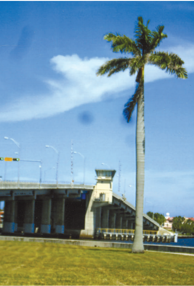
Opened in 1973, the 1,566 foot Lake Avenue Bascule Bridge is an engineering marvel. It has a 35 foot closed counterweighted span and a 90 foot horizontal opening. This is Lake Worth Beach’s third bridge.
