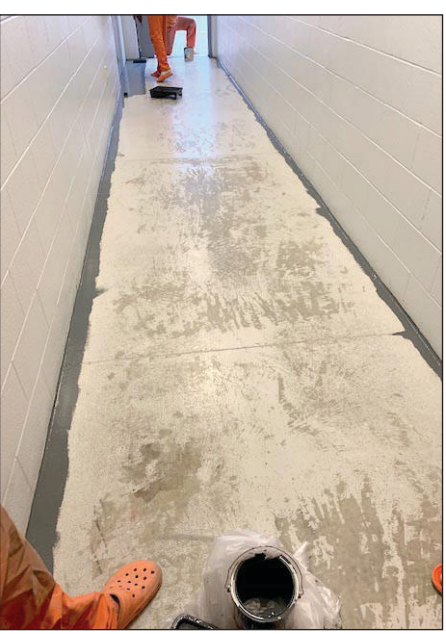
Before the hallway had a fresh coat of paint at RCDC.
