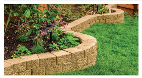
blocks or material should be positioned so that the joints are staggered for blocks, bricks or wood. A masonry blade will be needed to cut the harder materials; a circular saw will cut timber. Also, work against gravity by setting the second course slightly back from the first to help push back against the soil that is trying so hard to push forward. Repeat the process as each level is placed. Many retaining wall products are made with a lip to create this set back.
