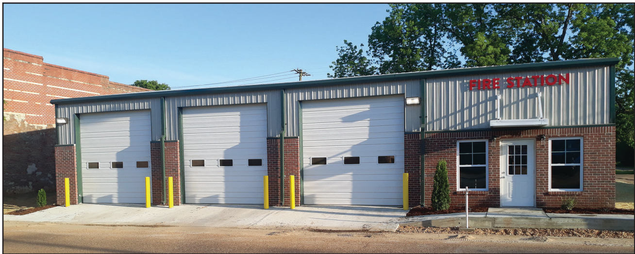
The town of Tchula got a new three-bay fire station approximately 3000 square feet with a training room and kitchenette. The station was built and financed by James Wessel, owner of Brindlee Fire Apparatus and Fire Truck Mall in Huntsville, Alabama. The station will be paid for by the fire rebate that Tchula receives each year from the insurance commissioner. MedStat the ambulance service for Holmes County will be on site and will provide service for the Tchula, Mileston, Thornton, Cruger and northern Humphreys County areas. Also, Tchula got a $6,033.00 grant from the Mississippi Department of Public Safety, the Division of Public Safety Planning, to buy body armor/bullet-proof vests, uniforms and flash lights for the police department. Officer Michael Rush found the source of the grant. Mayor General Vann filed the grant application and was assisted by Rush in gathering the necessary data to qualify. (Photo Submitted)
