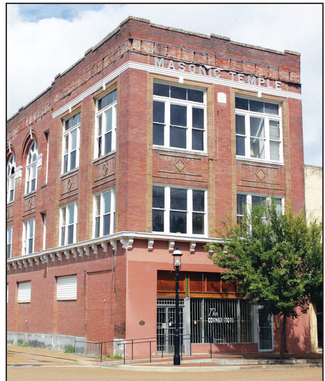
Pictured above, the three-story former Masonic Hall on the Lexington Court Square is currently having its roof rehabilitated after it collapsed in 2019.
