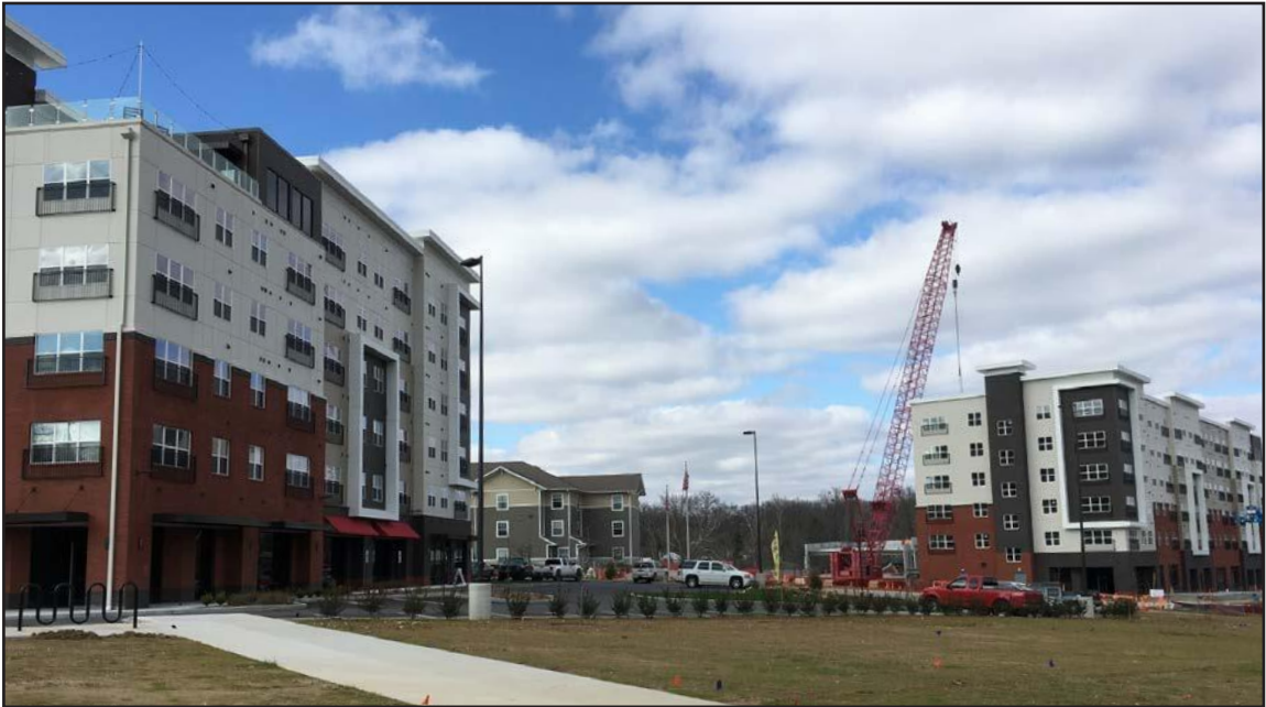
The two buildings that make up Whispering Heights in Edwardsville. The South Building, on the left, is finished. The North Building at right should be open in May. IBJ photo
