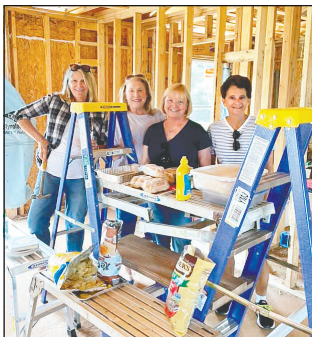
HELPING A NEIGHBOR — Future homeowner, Faith (not shown), was blessed by workers after her first wall went up at the Habitat build.
