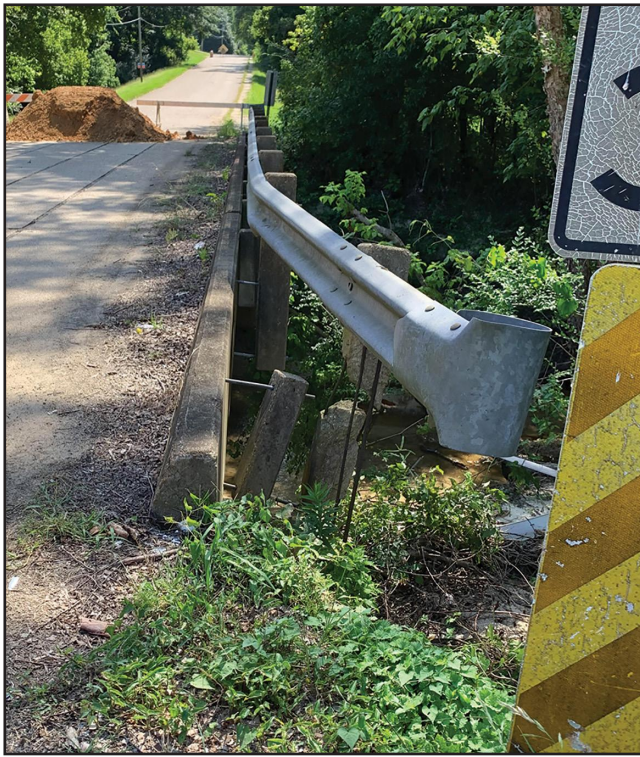
SCHOOL HOUSE BOTTOM BRIDGE
