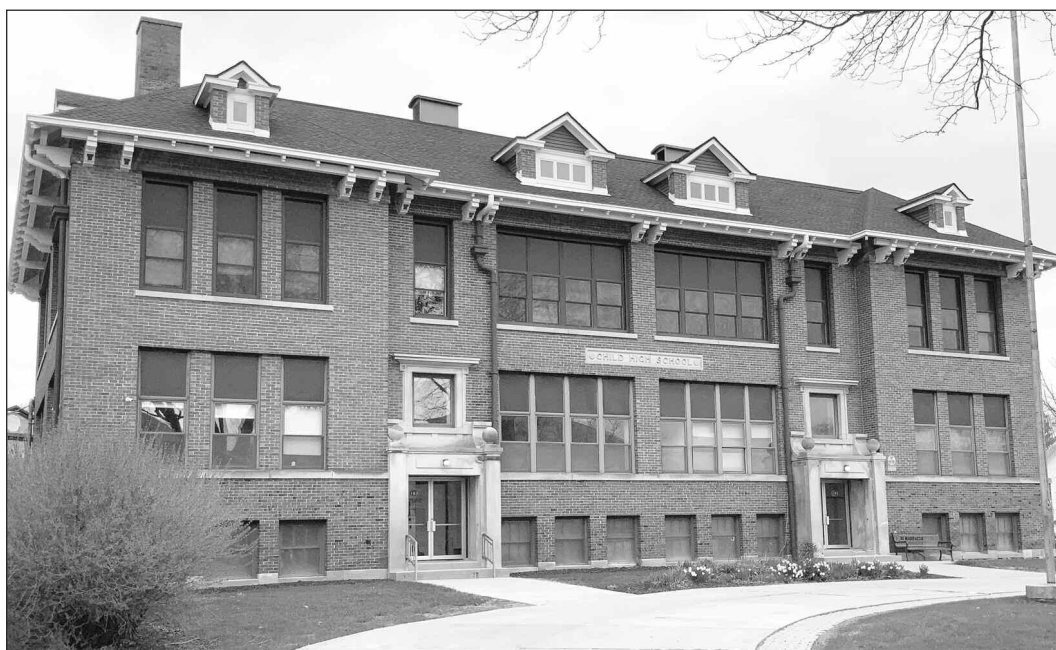
The former Child High School as it currently stands in Edgerton.
