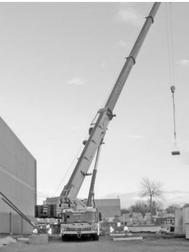
A crane begins the process of moving material from a stack and over the wall for use on a stair riser in the new auditorium.
