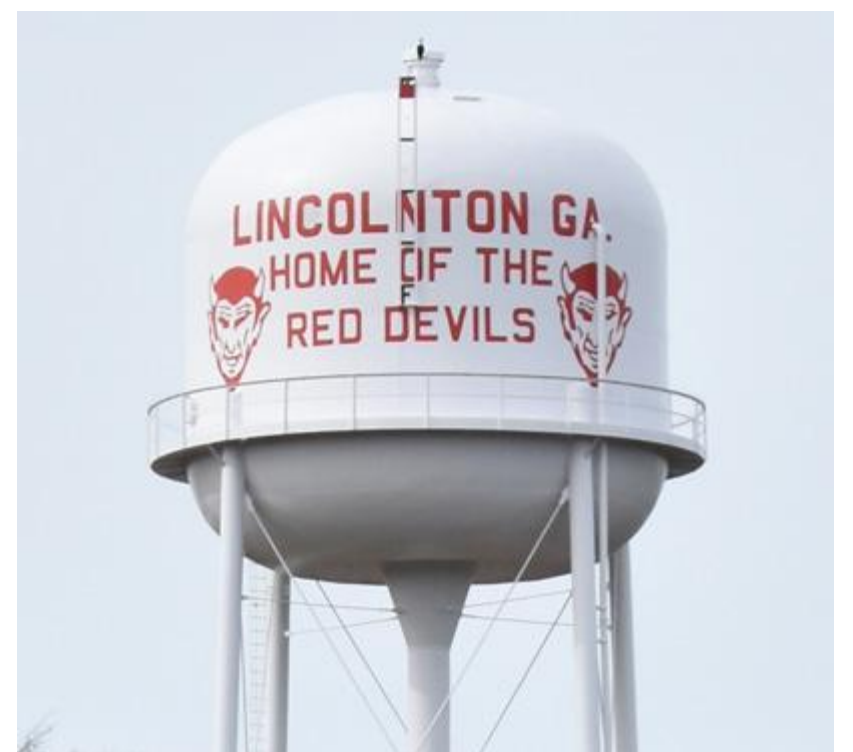
The refurbishment of the Drinkard Street water tank is complete including a fresh coat of paint on the "Home of the Red Devils" signage.
