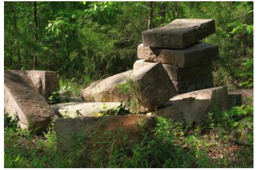
In Chester County at Landsford Canal you'll see the early 1800's handiwork of Irish stonemasons who crafted the canal's guardlock that lowered boats into the canal during floods. (Photos by Tom Poland).
