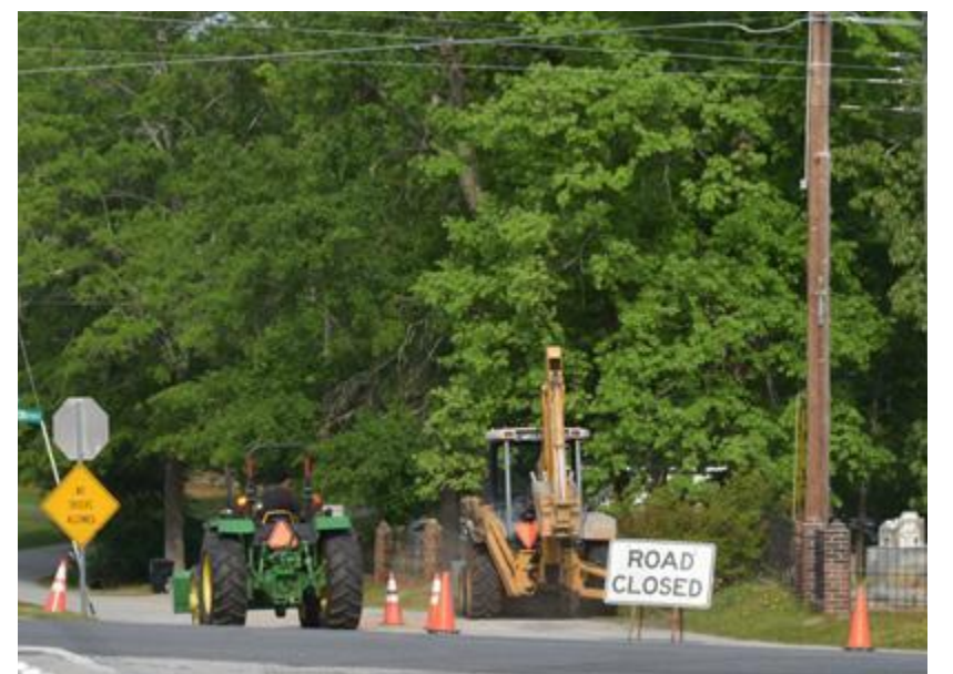
City of Lincolnton road crew recently completed repairs on Elam Avenue.
