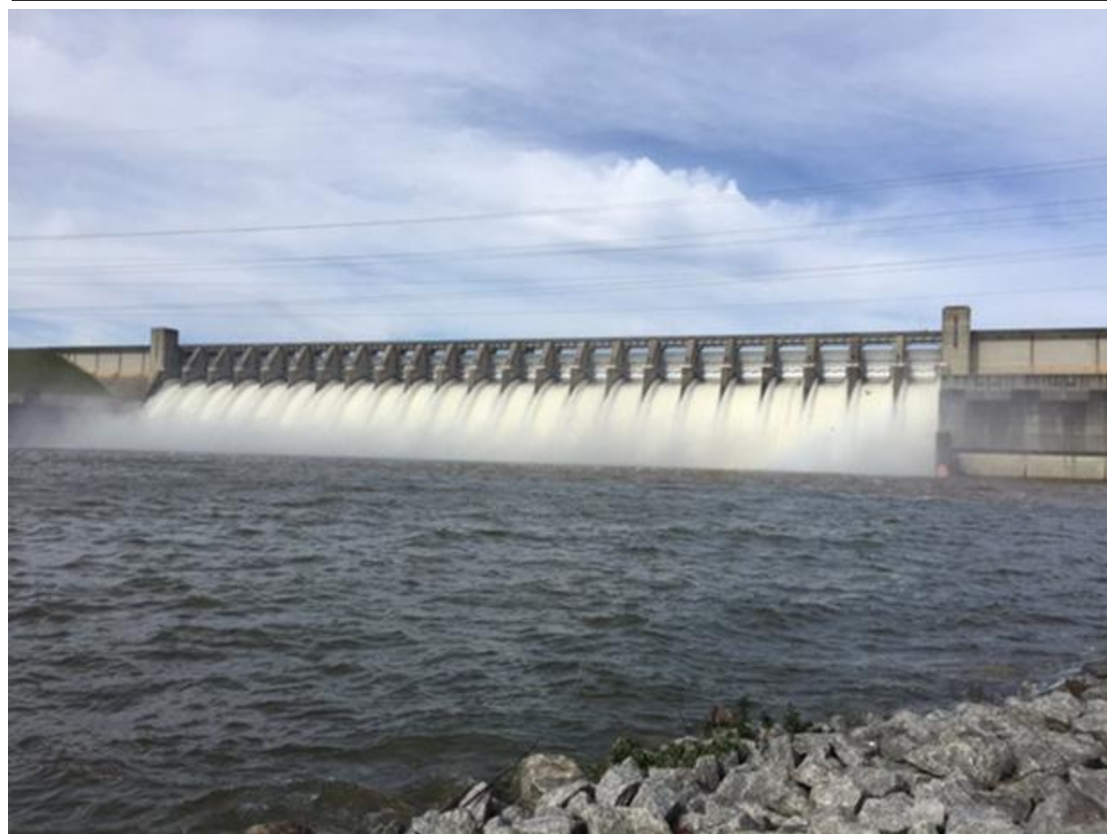
All 23 spillway gates at J. Strom Thurmond Dam were opened Wednesday, June 2, as a required safety test and to mark National Dam Safety Day which was May 31.
