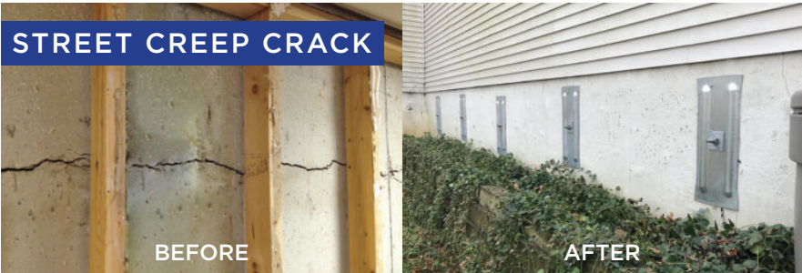
Wall anchors stabilize the foundation!
