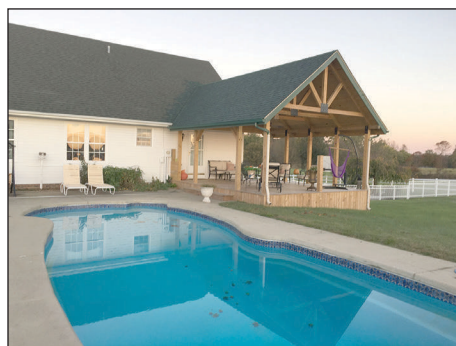
New deck before handrails.
