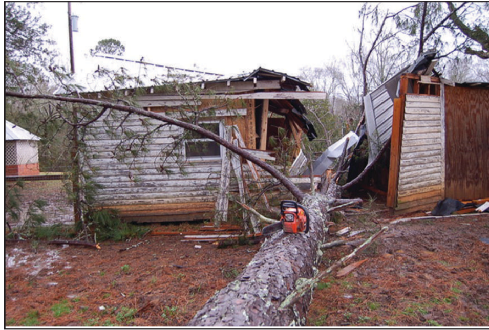
The Atwell's were awakened at 3:30 a.m. last Monday morning. Don went out to be greeted by this scene and their 36-year-old Appaloosa mare was trapped inside one of the buildings. He called 911, grabbed his chainsaw, and McCormick volunteers responded. -Don Atwell photo
