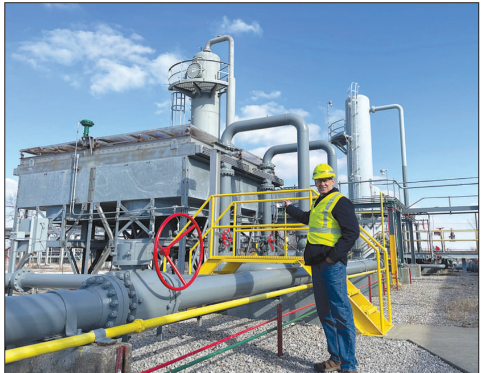
Steve Underwood, the director of gas storage for Ameren Illinois, at the Freeburg storage field. Enough gas is withdrawn there each winter to fill up Busch Stadium 83 times.
