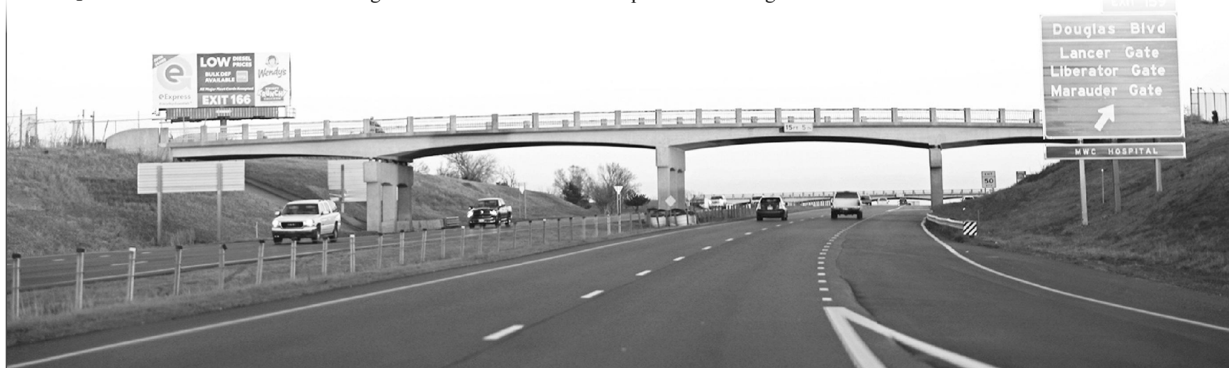
The largest single contract in ODOT history will soon result in a rebuild of the I-40 and Douglas Boulevard interchange as the interstate is widened. PHOTO BY KRISTIN HARRISON
