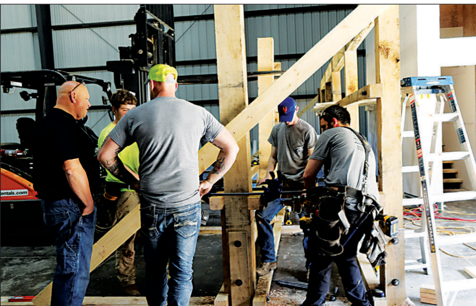
Junior Cecil, left, talks with Jason Thacker, facing away from the camera, while Thacker's crew works to install the first of the barrel racks in the rickhouse. The racks will extend several stories high and hold tens of thousands of barrels.
