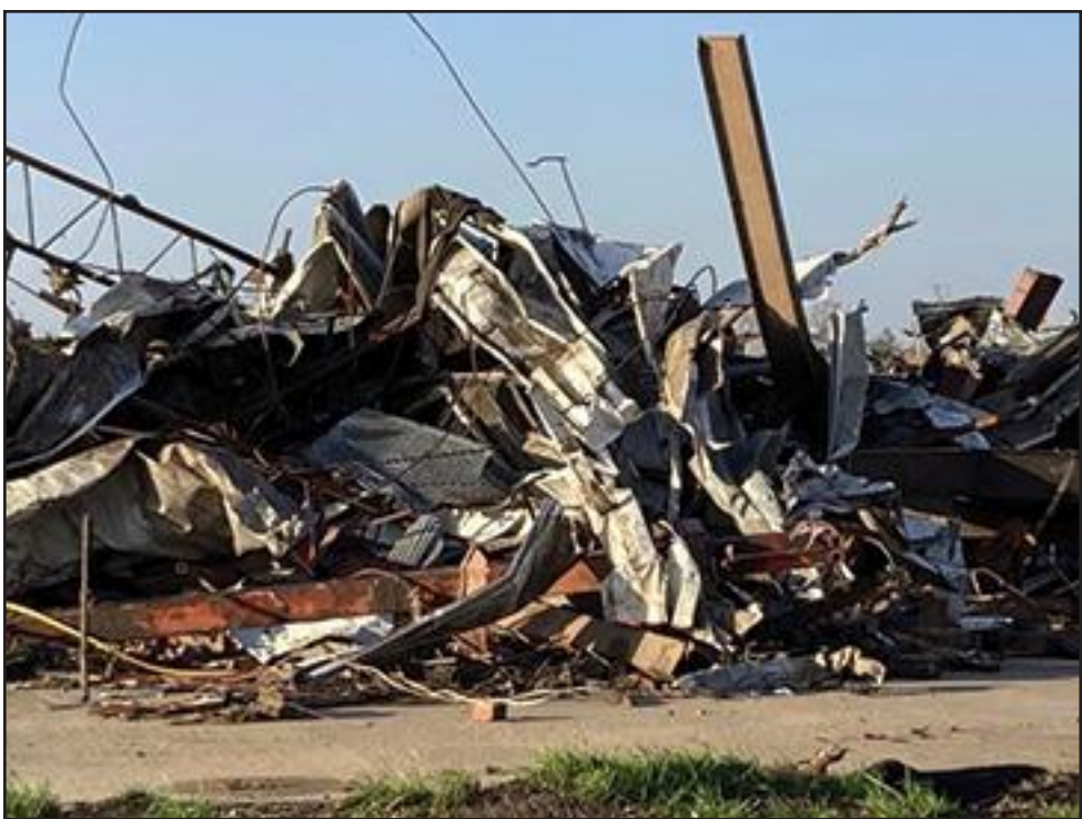
Debris covers a damaged structure in Rolling Fork, Miss., on Saturday. A powerful tornado tore through the Deep South on Friday night, killing several people in Mississippi and obliterating dozens of buildings. Rogelio Solis/AP
