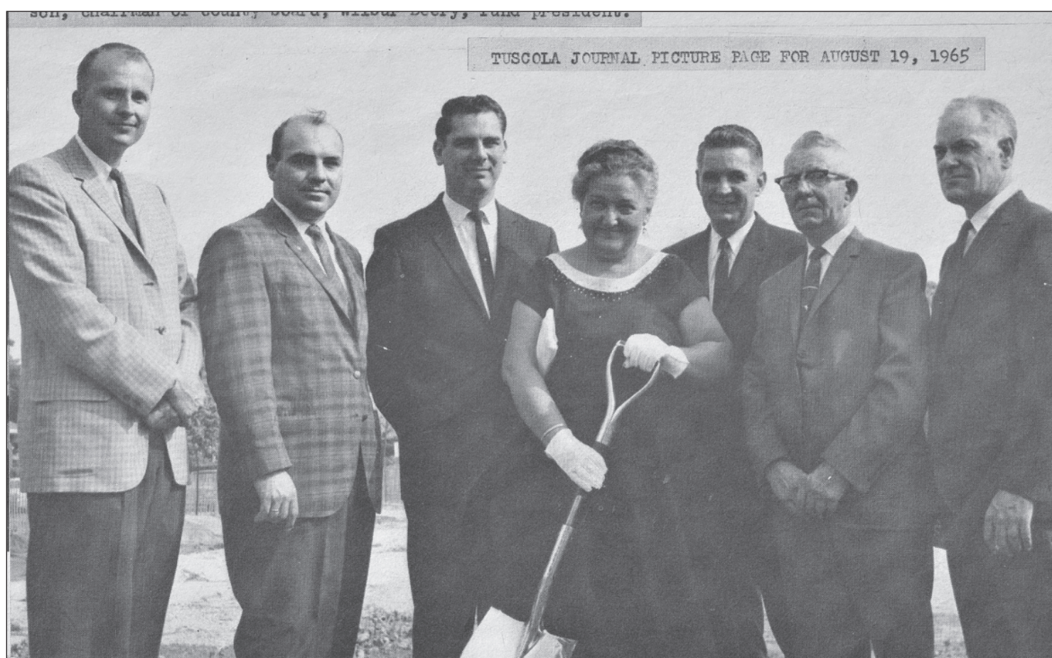
GROUND BREAKING for the "new" hospital in 1965. From left are William McCarty and Walt Jenkins, co-chairmen of the fundraising steering committee, Max Kersbergen, hospital administrator, Mrs. Harry L. Pate, president of the hospital auxiliary, the Rev. John Jones, fund treasurer, Marion Stephenson, chairman of the Douglas County Board, and Wilber Beery, fund president.
