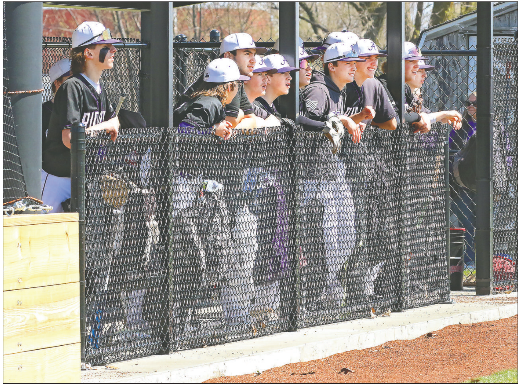
THE ARCOLA BASEBALL TEAM is getting settled into the new dugout facilities while watching Martinsville warm up before the first official home game of the season. The totally new dugout areas are just part of the renovations to the baseball field at Moore Park. The city of Arcola continues to work on the baseball, softball and t-ball diamonds in addition to several other improvements being made at the park. Arcola won the home opener against Martinsville 21-2 on Saturday, April 8. Photo by Nancy Raiden.
