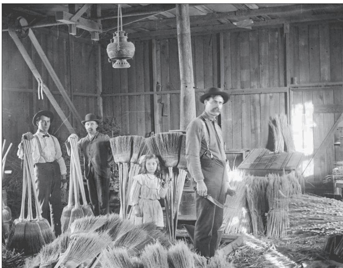
THERE WERE SEVERAL broomcorn companies in Arthur. In 1894, D.L. Fishleigh went into this business with warehouses on both railroads.
