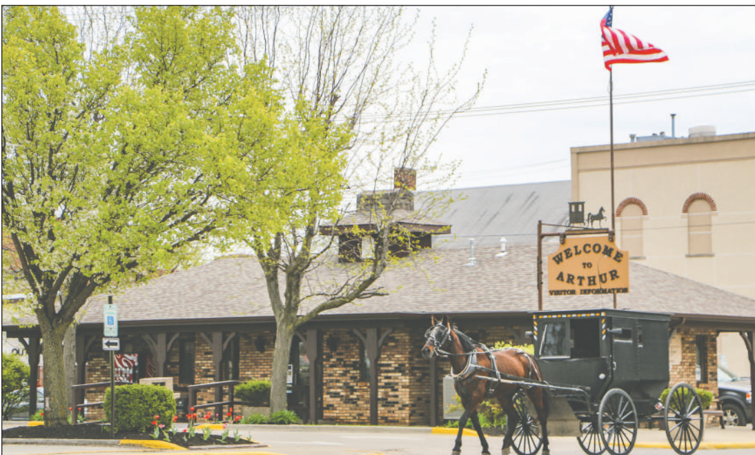
Construction for Arthur's Welcome Center (then called the tourist center) began in 1973.
