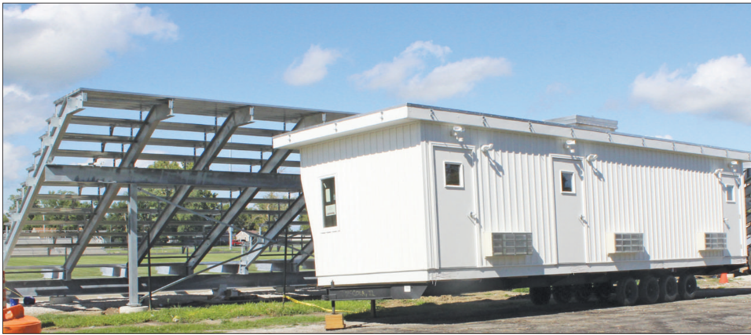
THE NEW PRESS BOX for Tuscola High School's football field and track has been delivered and is expected to be installed on top of new bleachers this week. Photo by David Porter.
