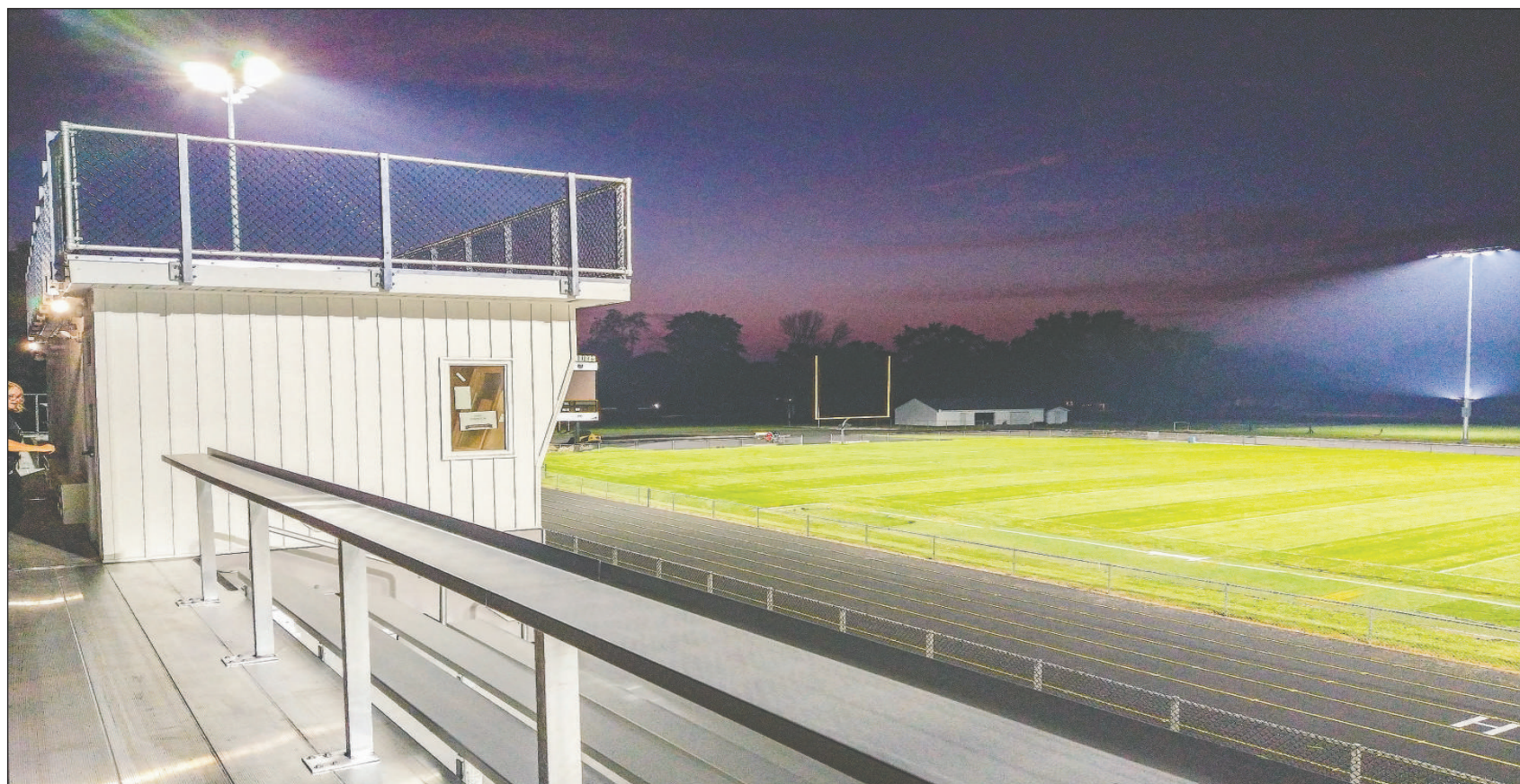
THIS VIEW was taken Monday evening from the middle of the east tier of new bleachers at Tuscola High School. Spectators there will be able to see only a small part of the school's new, $250,000 scoreboard. The view worsens as one moves west toward the press box. Stan Wienke, former head football coach, addressed the School Board Monday to outline deficiencies in the improvements. Photo by David Porter.
