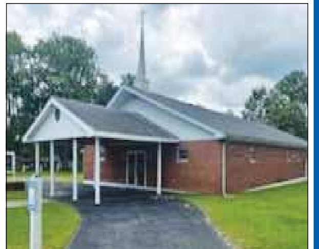
Covered entry way, 3000 sq ft church. Garden shed included. Selling "as is". $200,000 109 College Street, Alhambra
