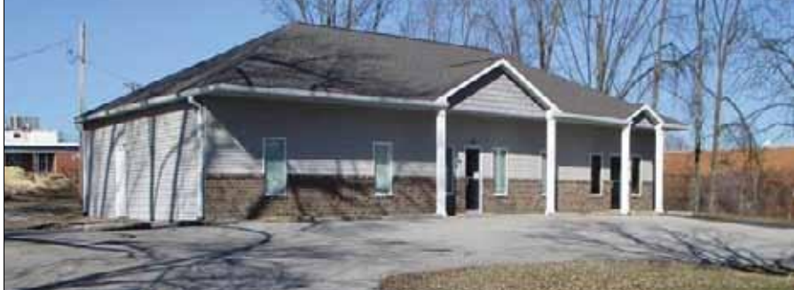
Well known Professional Retail building on Walnut High traffic area. 206 Walnut Street, Highland- $460,000
